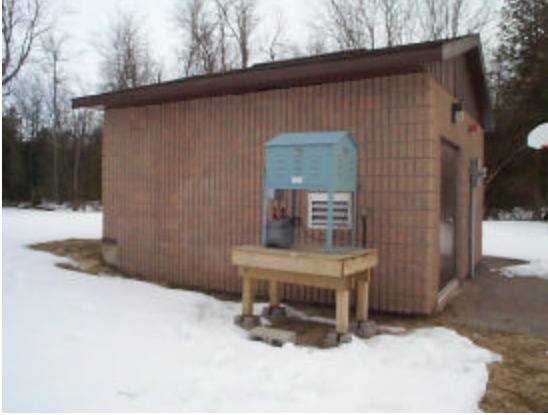
Scott Point Air Sampling Station
